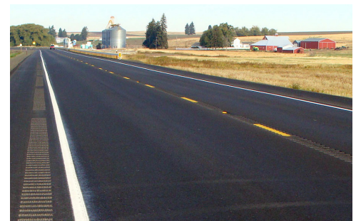
Shoulder rumble strips and center line rumble stripes are installed on this roadway. Source: FHWA
