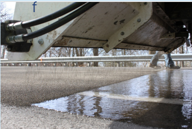
Automated application of HFST. Source: FHWA
