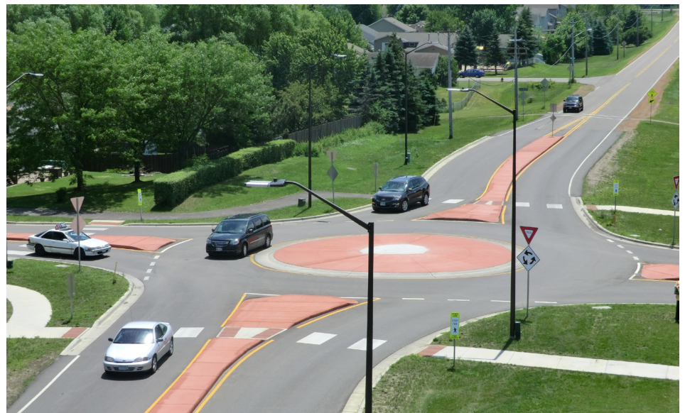
Example of a single-lane roundabout. Source: FHWA
